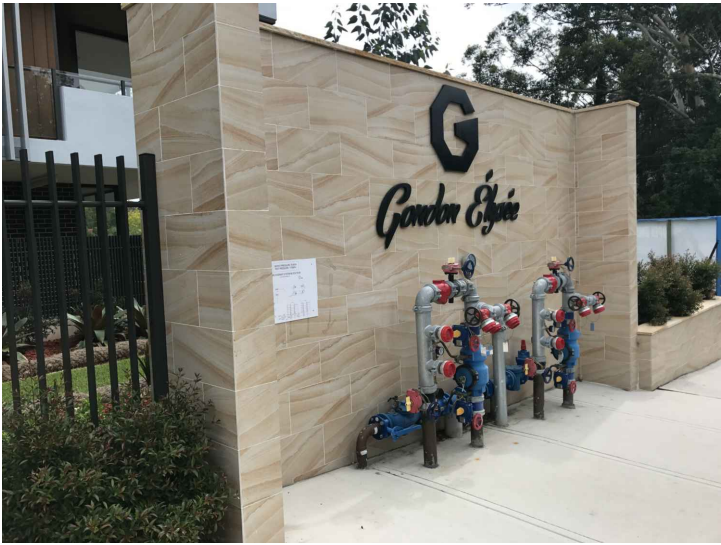
SIGN VIEWED FROM FOOTPATH TRAVELING NORTH. A
